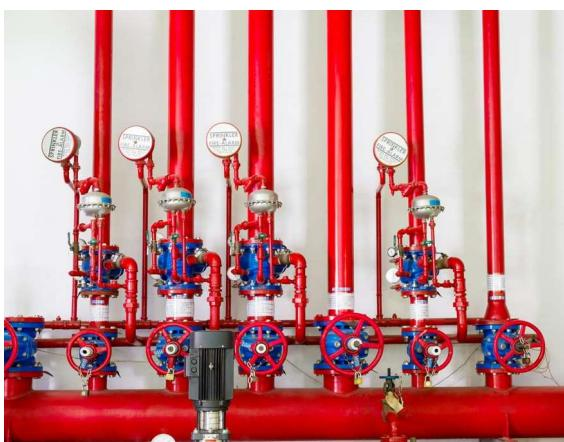
An automatic sprinkler system is intended to detect, control and extinguish a fire, and warn the occupants of occurrence of fire. The installation comprises fire pumps, water storage tanks, control valve sets, sprinkler heads, flow switches, pressure switches, pipe work and valves. The system operates automatically without human intervention.
