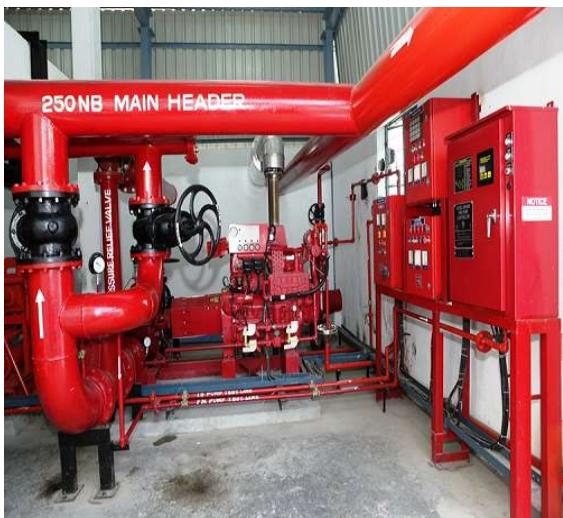
Fire hydrant installation consists of a system of pipe work connected directly to the water supply main to provide water to each and every hydrant outlet and is intended to provide water for the firemen to fight a fire. The Fire Hydrant Line is always kept pressurized with water. A fire-fighter connects a fire hose to the fire hydrant and releases a valve to get water from the water main.
